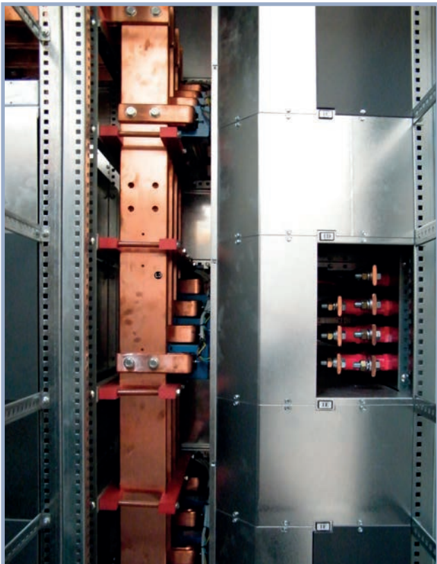
Forma 4b (in manutenzione) Form 4b (during maintenance) Forme 4b (pendant manutention)
